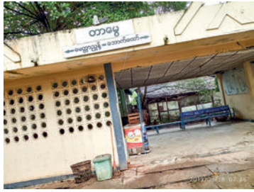
The photo indicates the Tamway Station that is included in the station upgrading project.
