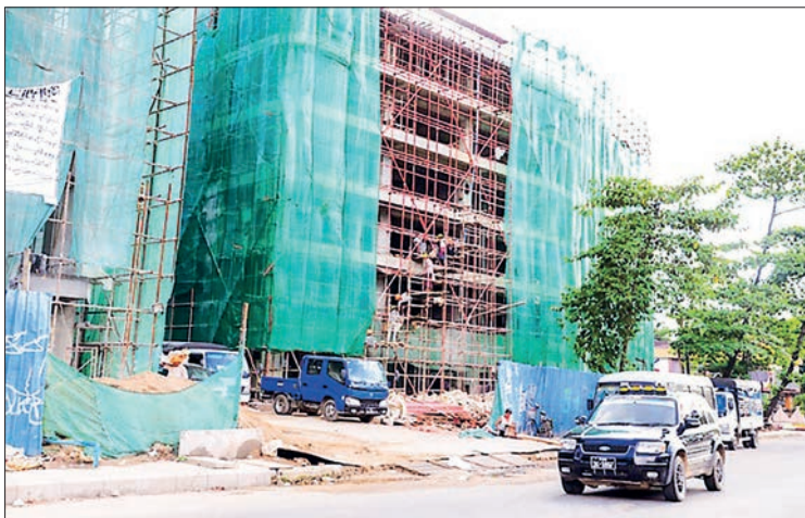
A building is seen under construction in the Yangon Region.
