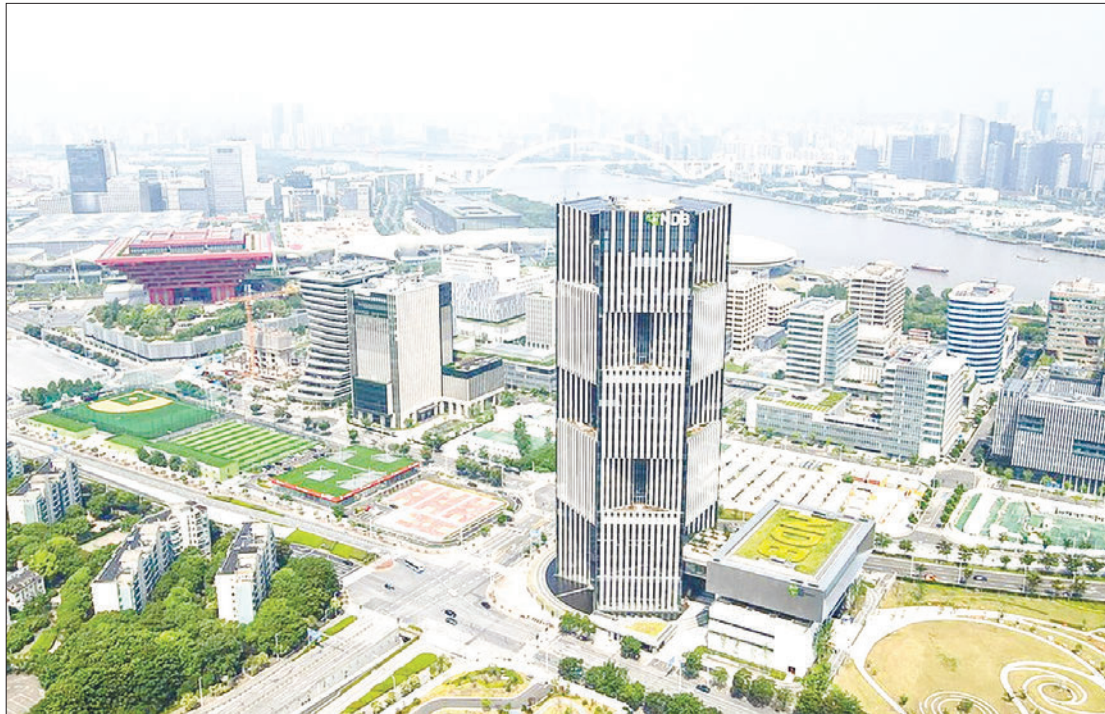
Aerial photo, taken on 17 June 2022, shows the headquarters building of the New Development Bank (NDB), also known as the BRICS bank, in East China's Shanghai. PHOTO: FANG ZHE/XINHUA
