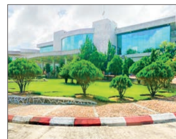
The Ministry of Commerce Office building in Ottarathiri of Nay Pyi Taw.
