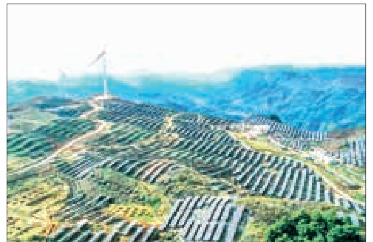
This aerial photo taken on 16 November 2023 shows the Dingdongpo wind power-photovoltaic project in Shiqian County of Tongren City, southwest China's Guizhou Province. With a combined power-generating capacity of 100,100 kilowatts, the Dingdongpo wind power-photovoltaic project has been successfully connected to the grid. PHOTO: XINHUA
