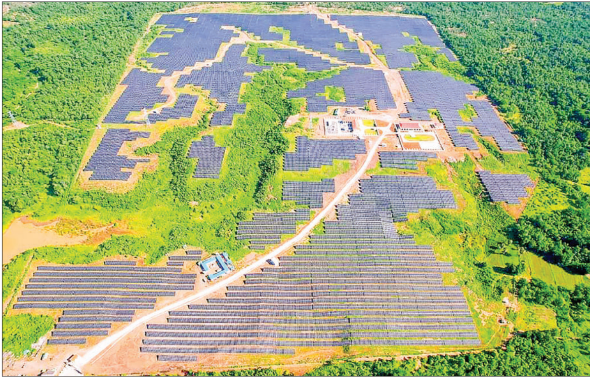
An aerial panoramic view shows a site of the solar power station project.
