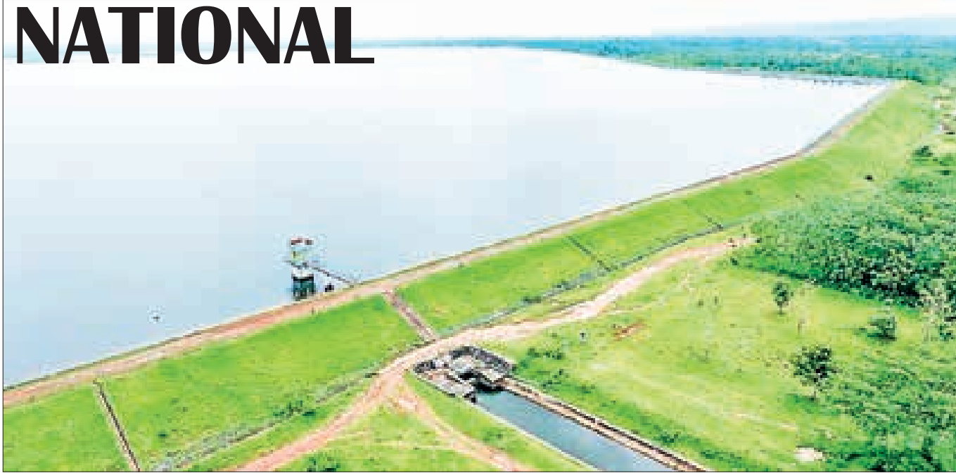
The Yebok Dam in Hlaingbwe Township supplies agricultural water to 1,192 acres of monsoon paddy.
