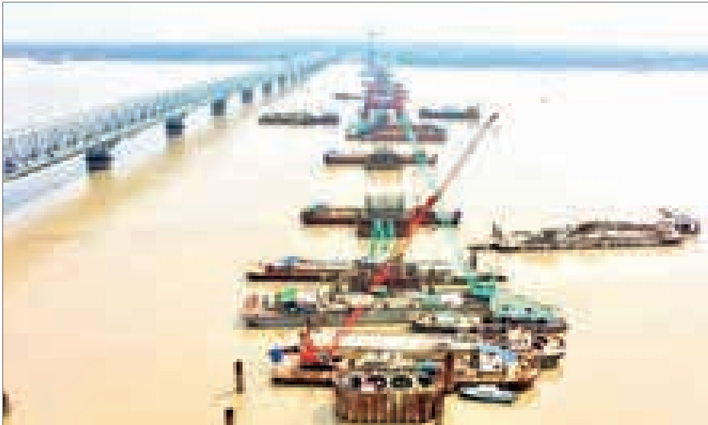
Panoramic Progress: Construction of the Thanlyin Bridge 3 over the Bago River unveiled.
