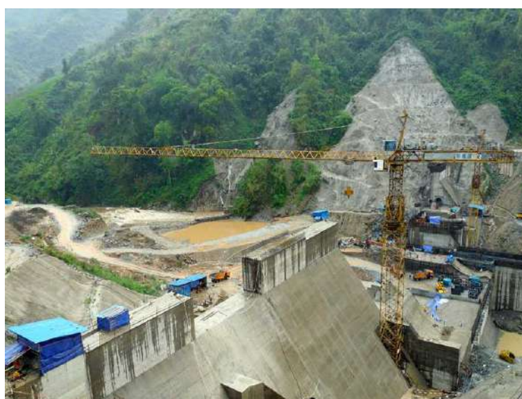
Fig. 12. Dam construction on the Chibwe river by China Power Investment. Photo: Frank Momberg, April 2010.
