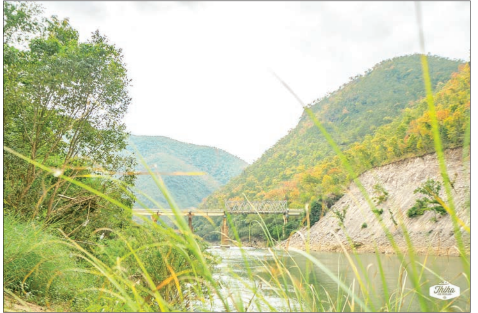
Dutthawady River Bridge
