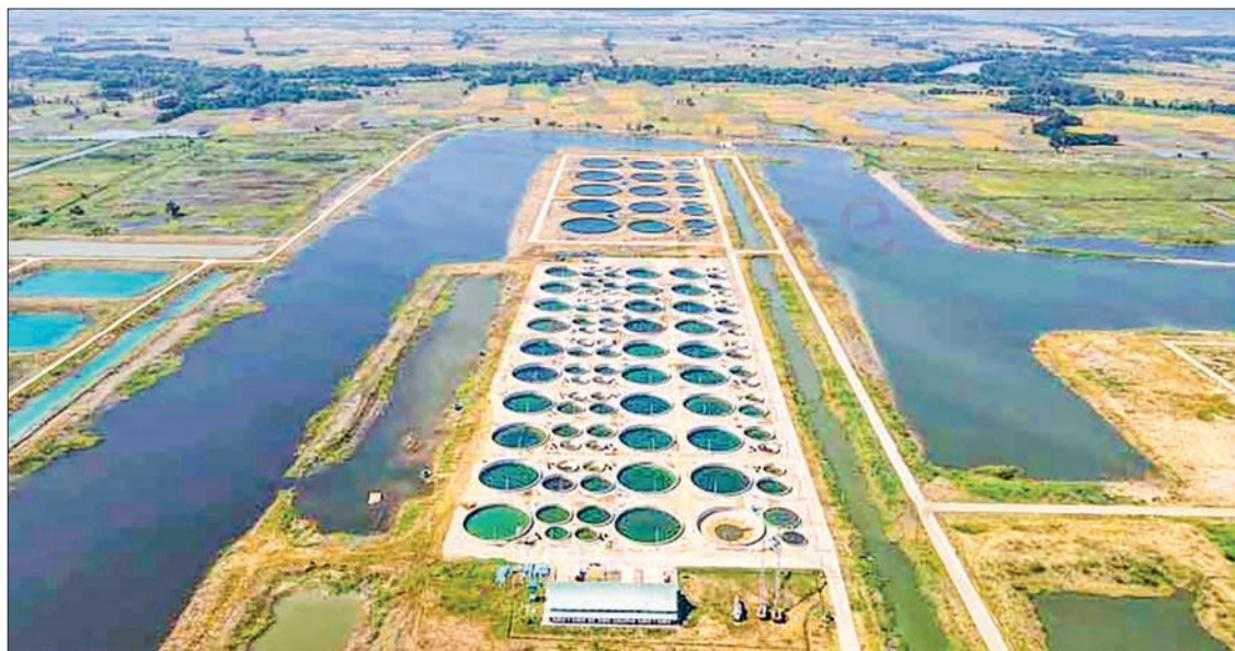
General view of the fish farming in circular tanks.
