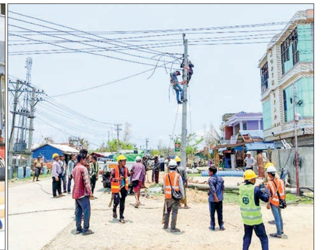
Electricians repairing power cables to supply electricity to locals in Yathedaung.
