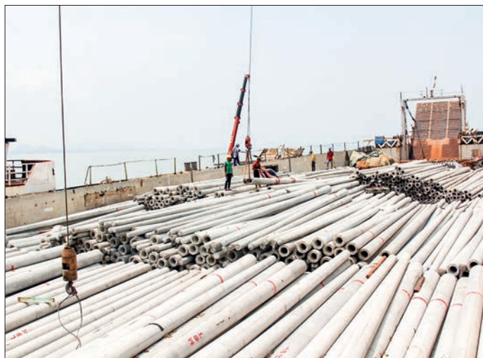
Unloading of concrete lamp-posts
