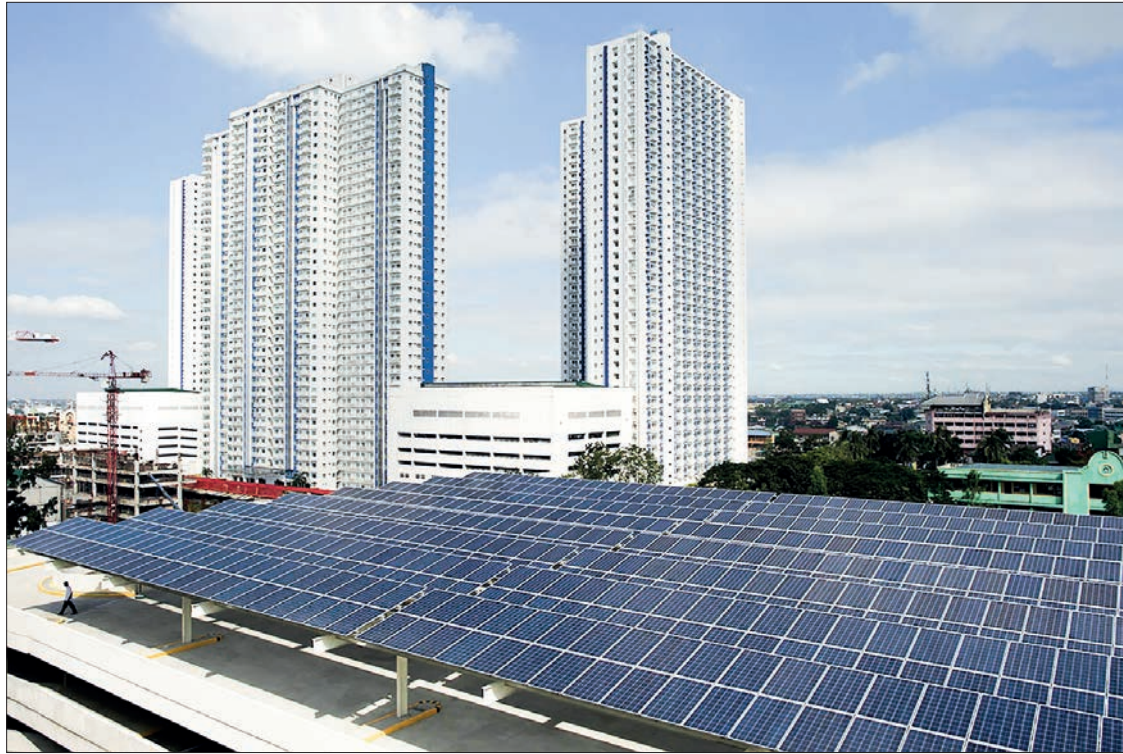
The solar panels at the roof deck of a mall in Manila. PHOTO: REPRESENTATIVE IMAGE/ NOEL CELIS/ AFP
