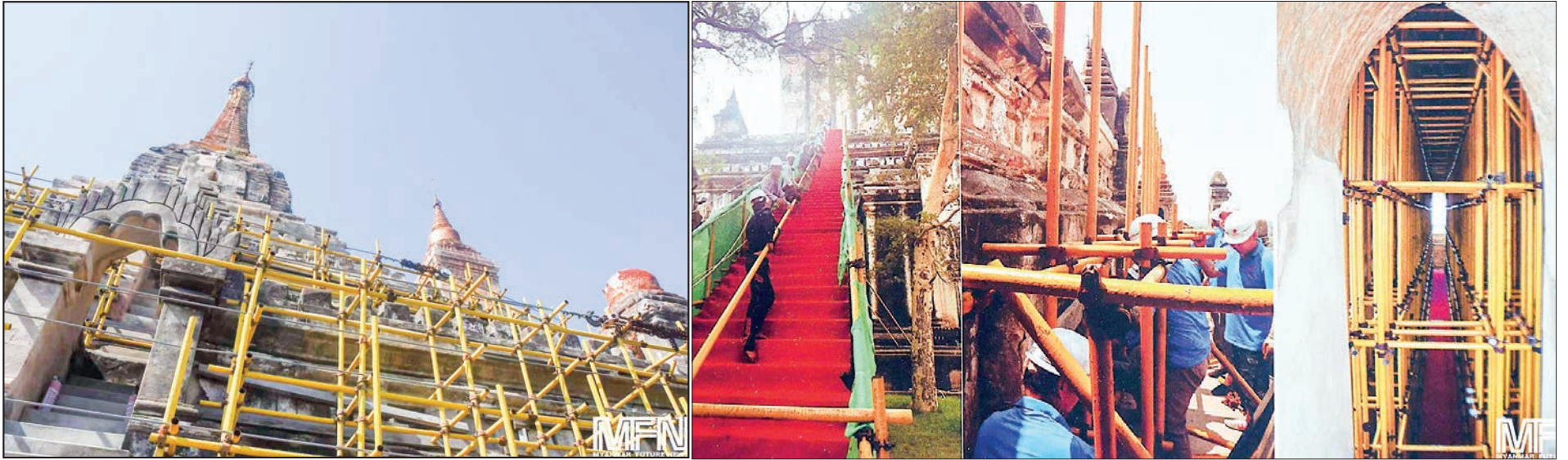
The Thatbyinnyu Temple is seen under maintenance and restoration.
