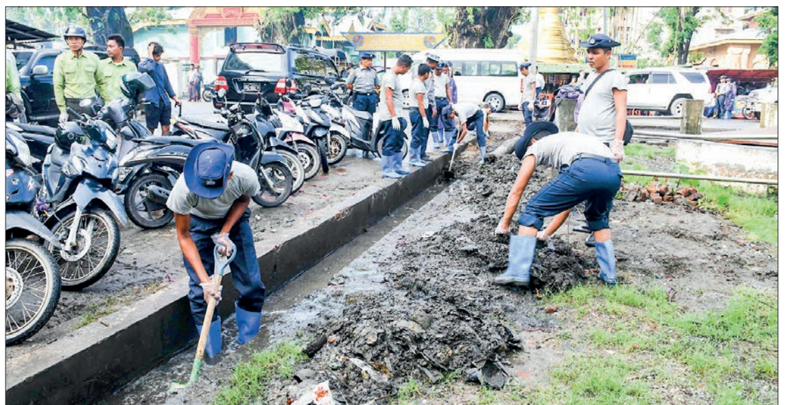
The drainage improvement works in progress in Sittway on 8 July 2023.
