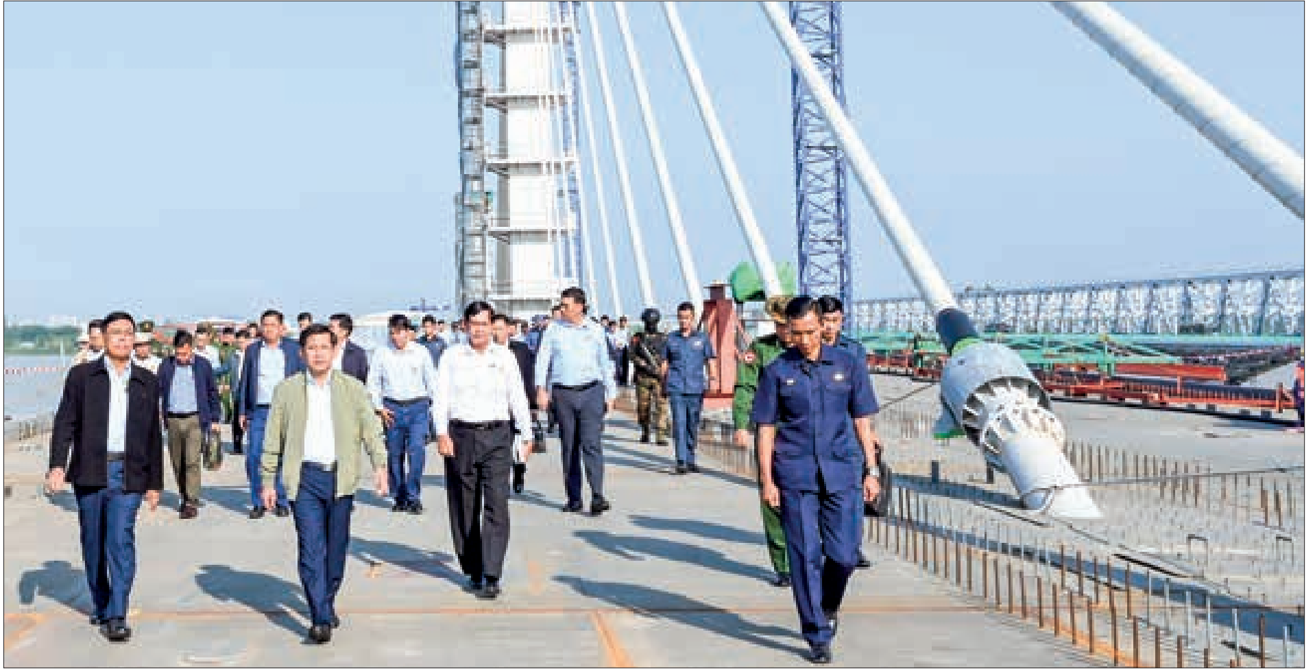
Chairman of the State Administration Council Prime Minister Senior General Min Aung Hlaing inspects the progress in construction of Bago River Bridge (Thanlyin Bridge-3) in Yangon Region yesterday.
