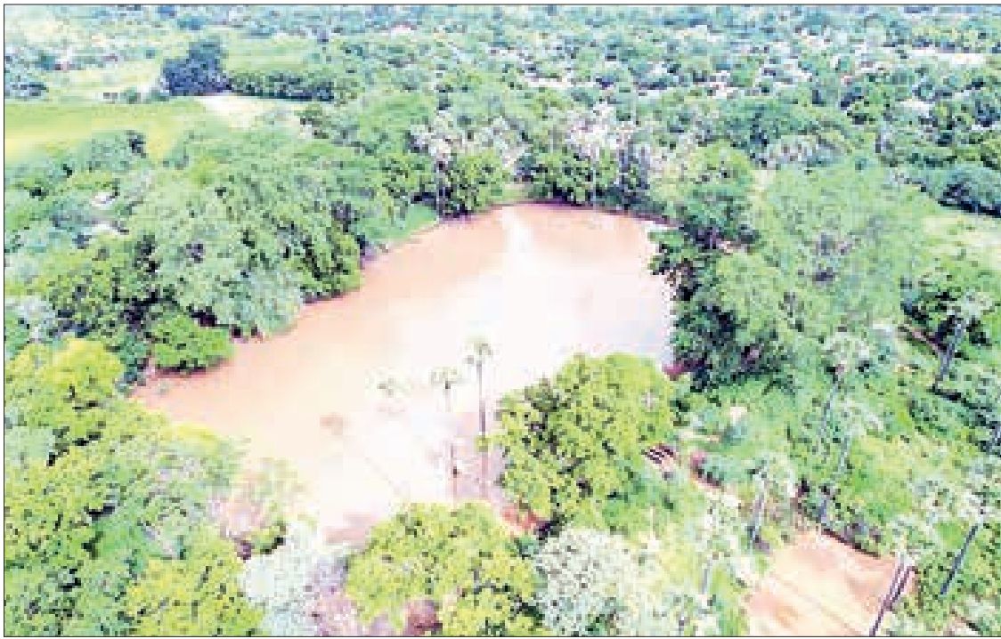
Excavation and renovation processes of ancient lakes.
