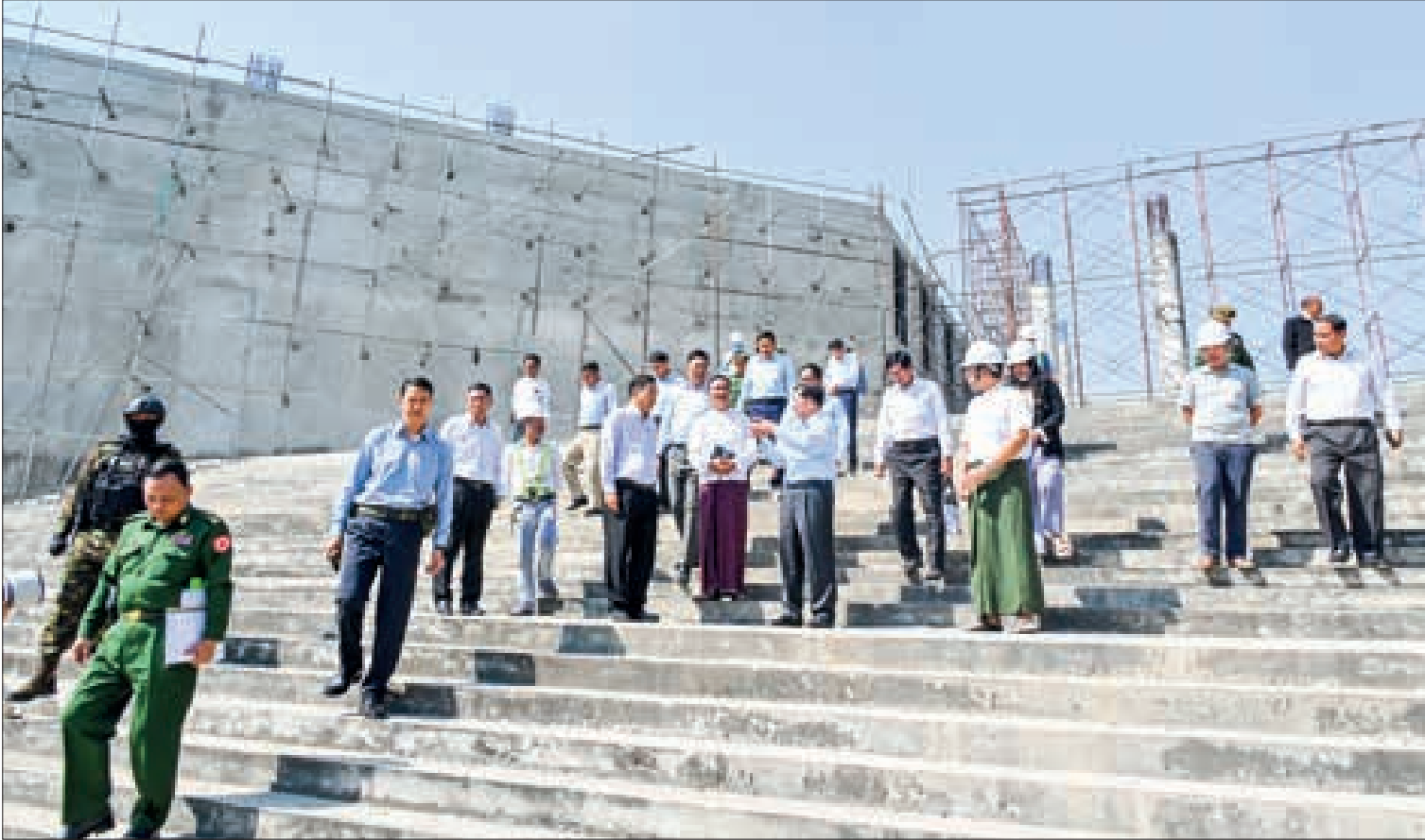
Chairman of the State Administration Council Prime Minister Senior General Min Aung Hlaing looks into the progress of the three-storey lecture hall being built on Yangon Western Technological University campus in Hlinethaya Township of Yangon Region yesterday.
