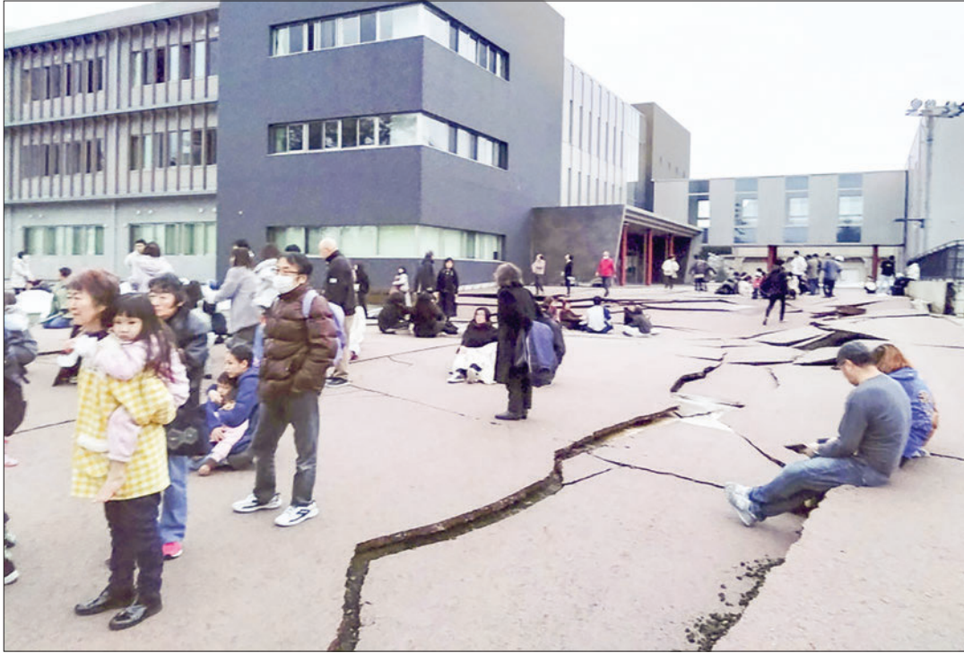
Large cracks are seen on the ground in Wajima, Ishikawa Prefecture, on 1 January 2024, after a strong earthquake rocked a wide area on the Sea of Japan coast in central Japan. PHOTO: KYODO
