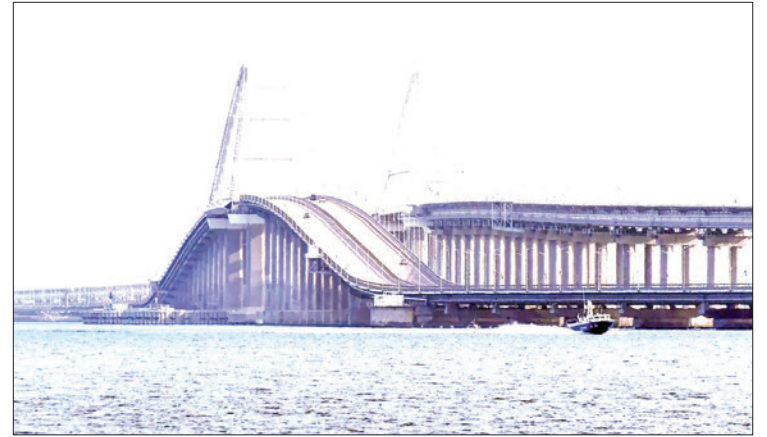
Left side of the Crimean Bridge opened for traffic. PHOTO: SPUTNIK
