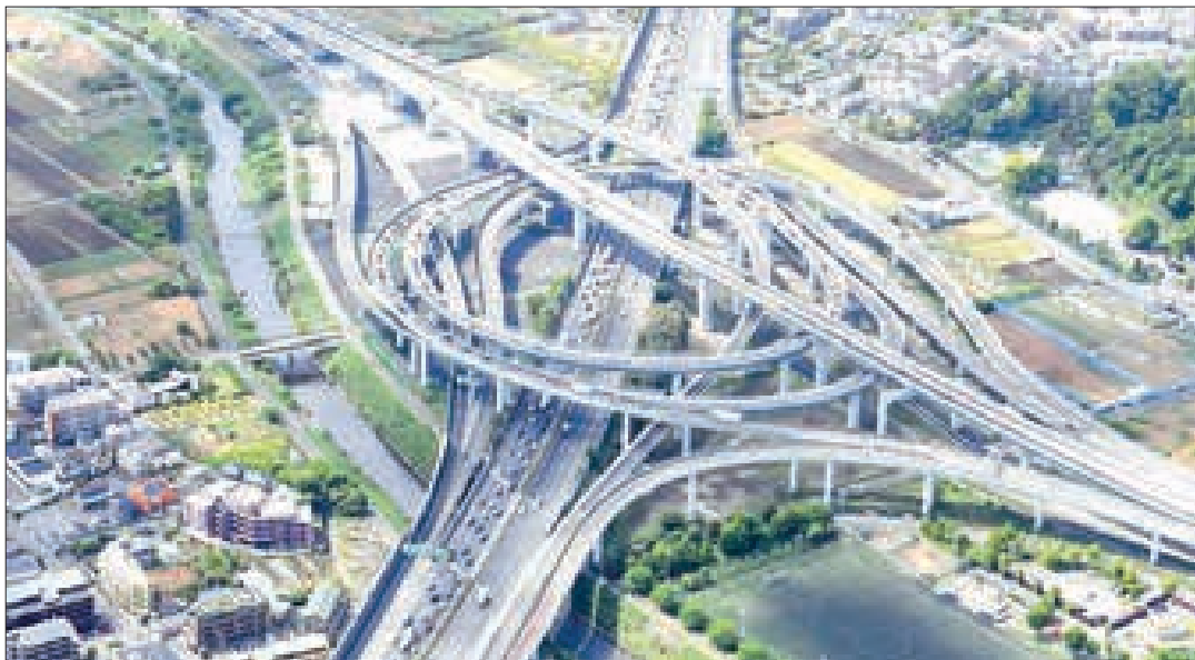
This expansion, covering road and railway transport, as well as the forestry and timber sectors, marks the first since the programme's inception in 2019. PHOTO: KYODO
